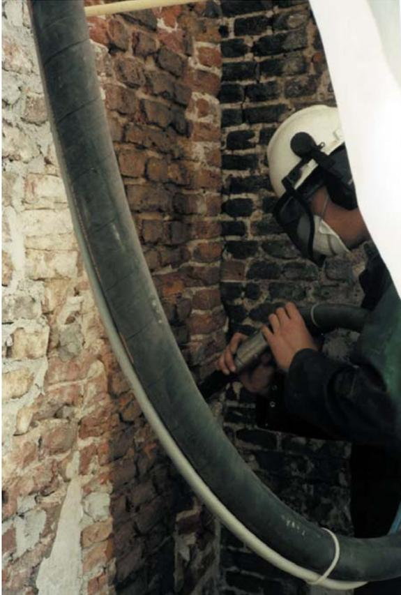
During a Gorinchem, Netherlands building renovation, the contractor was required by the building architect to selectively remove heavy deposits of creosote, pitch and lignum from the main chimney. The contractor chose Brown Sponge Media™ abrasive in place of wet blasting or hand-tooling to remove the contaminants from the chimney. The contractor made the choice based on the location and age of the chimney and the Sponge Blasting technology characteristics:
