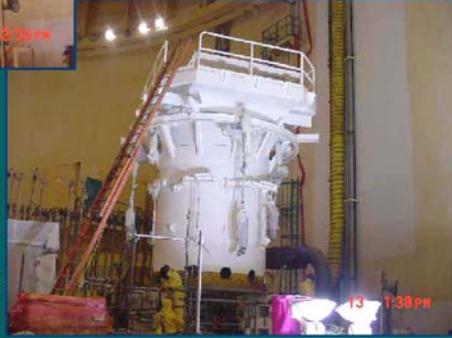
After Sponge Jet-Blasting and Painting
