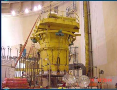
Before Sponge Jet-Blasting and Painting
